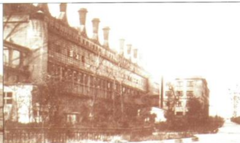
Новомосковская ГРЭС Novomoskovskaya Power Station
