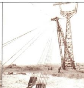
Монтаж опор ЛЭП (50-60 гг.) Erection of supports of power transmission lines (50-60-ties)
