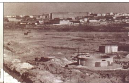
Начало строительства ТЭЦ-23 Construction of TEP-23 has commenced
